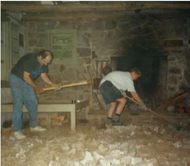
September 1995 - Steve Babor and Dan Barham breakup and remove the original cabin floor
