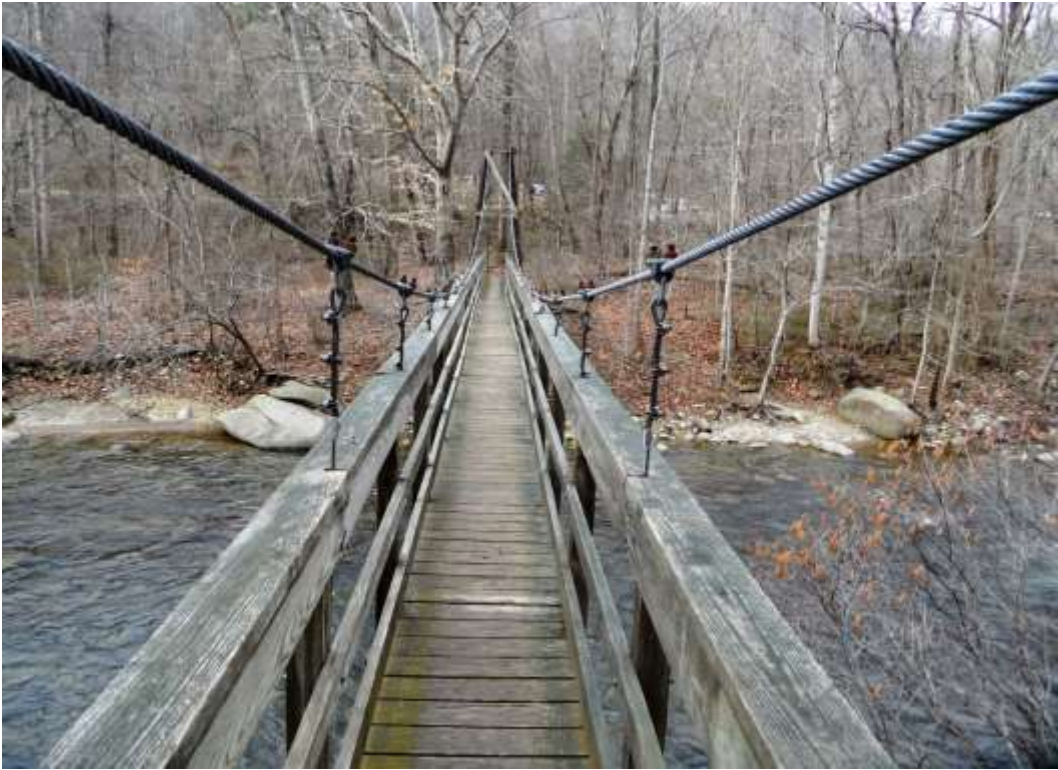
Tye River Bridge - 2012
