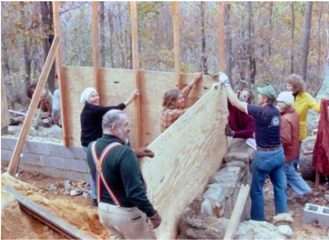
November 1979 - Foundation Work - cinderblock foundation is visible as we erect plywood - Left to Right - Margaret Crate, Gene Krah, Bob Adkisson, and Otey Shelton with hammer
