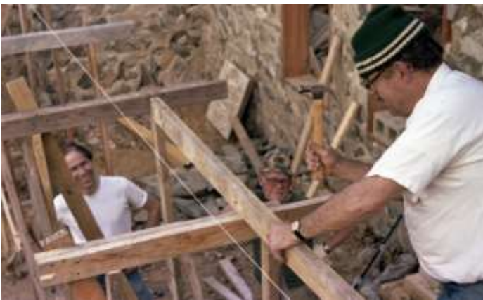
Mal Higgins and Gene Krah work on temporary interior scaffolding , Late Summer 1981
