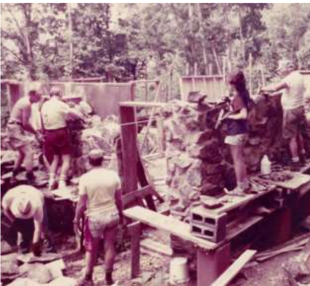
Summer of 1980 - Large Group of Workers lay rocks as the 4 cabin walls slowly rise
