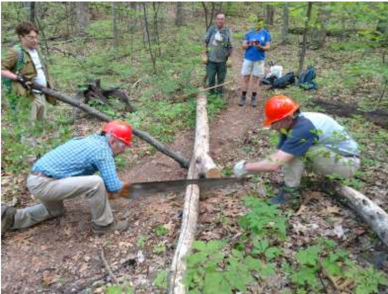
John Sima uses a lever to assist as others cut a tree fallen across the trail
