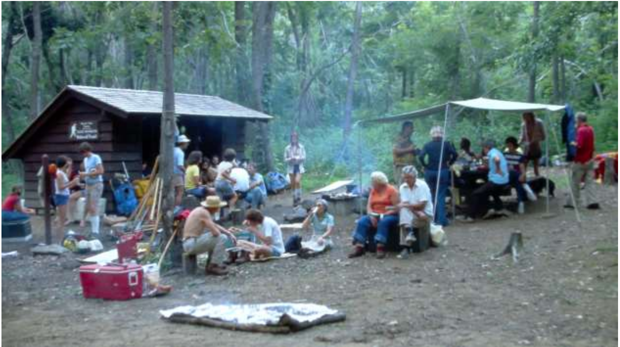
July 1978 - Mau-Har Trail Construction
