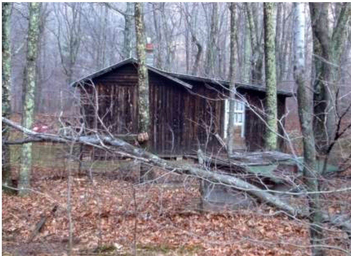
April 1990 - Backside of Campbell Cabin at Maupin Field Gap With a dog kennel and some fencing visible
