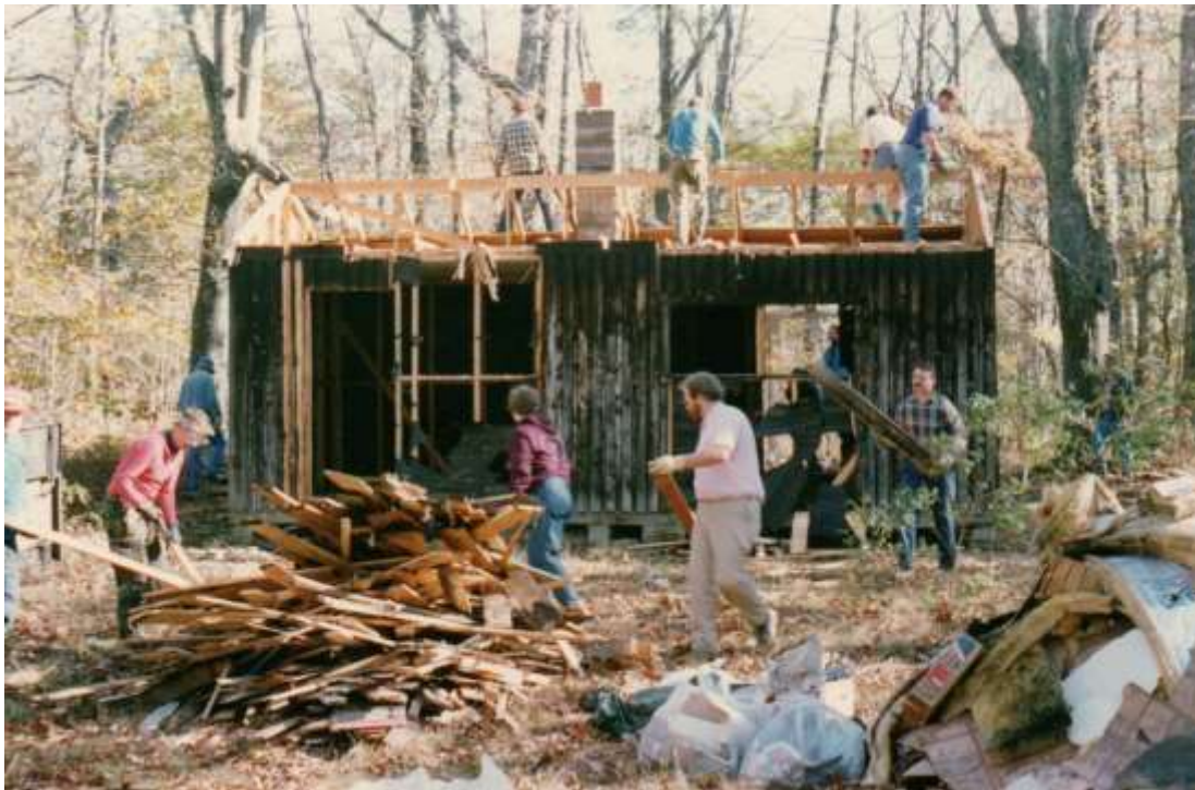
Tearing down Campbell Cabin at Maupin Field - 1990
