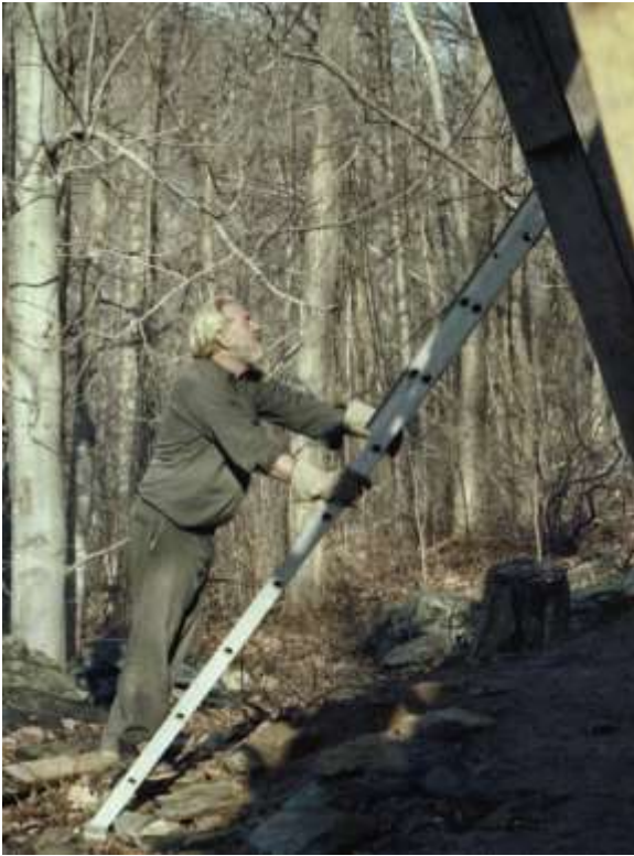
Curtis Eley on ladder building the Cabin 1982
