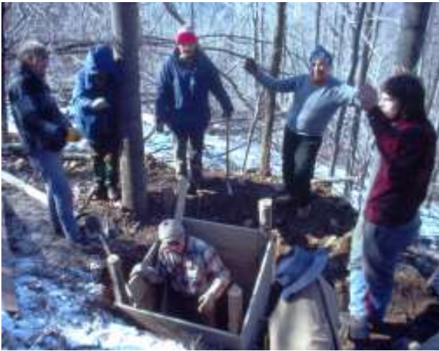
February 1979 - One of the first jobs at the cabin site - dig a hole - build an outhouse - Bill Newsom and Steve Crate - right side
