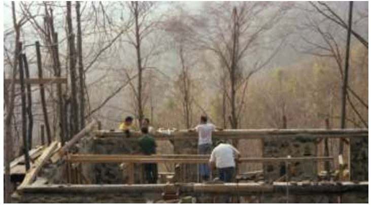
Cabin Walls going up 1981
