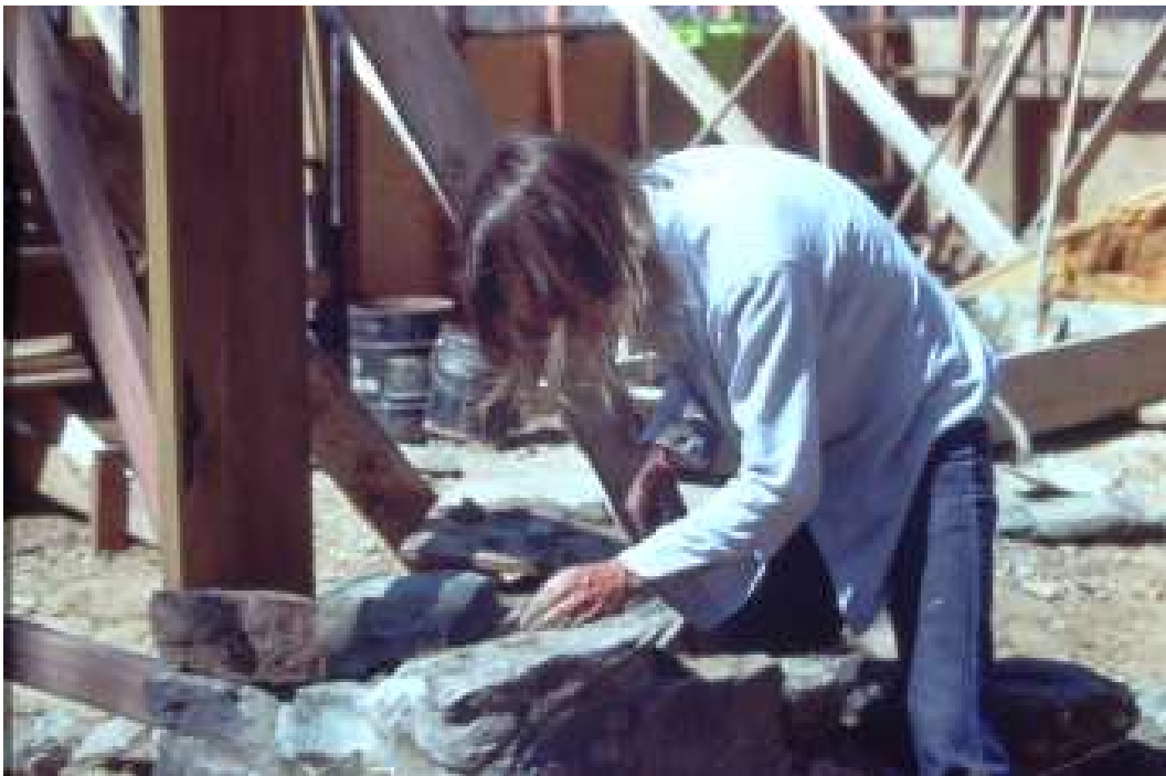
April 1982 - Bob Adkisson – laying stones at one of the corners
