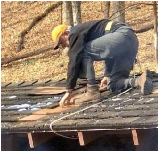
Milton Beale repairing Harpers Creek Shelter Roof
