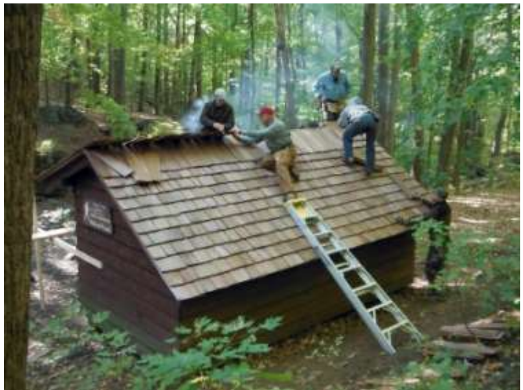
Harpers Creek Shelter gets a new roof
