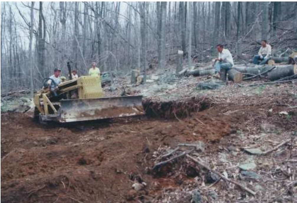
Bulldozing Cabin Site Clearing
