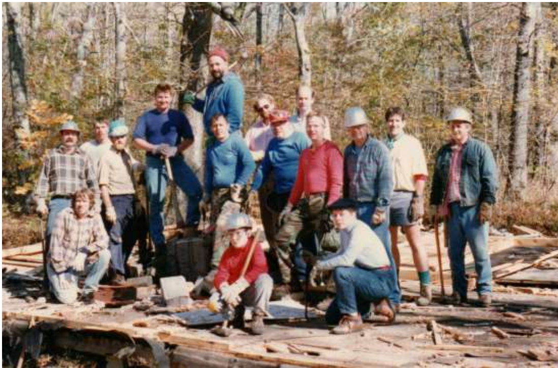
Campbell Cabin Demolition Crew - 1990
