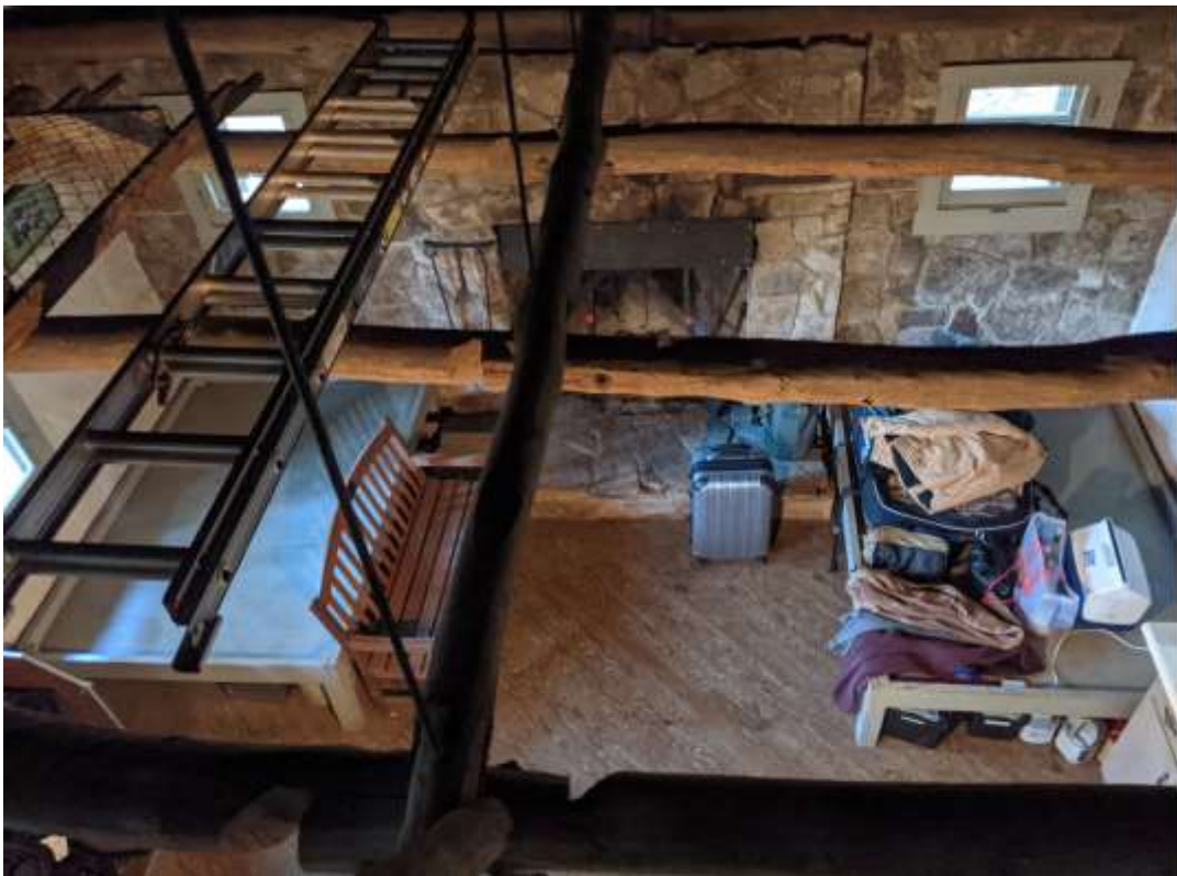
Looking down at one end of the cabin from the loft
