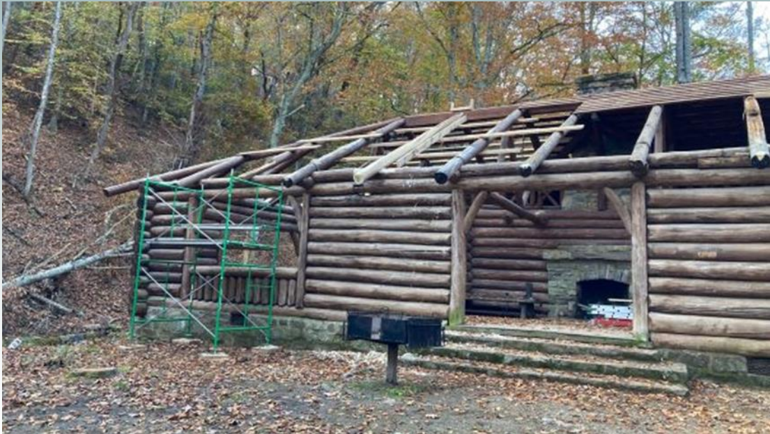
New rafter installation
