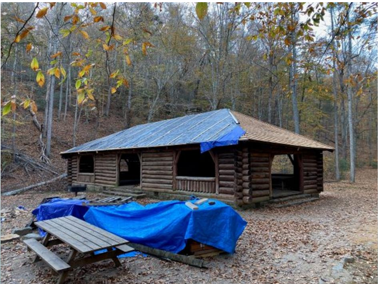
Tarps installed on north side.
