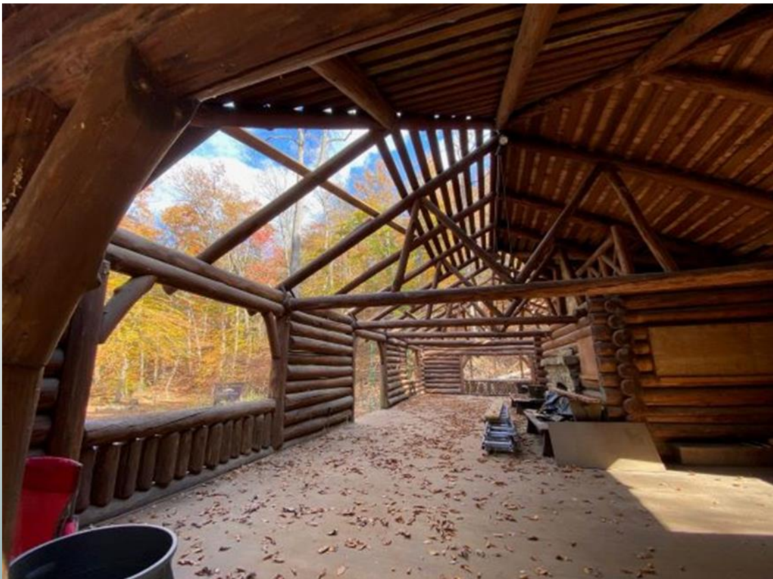
Before the purlins were replaced (early November session).
