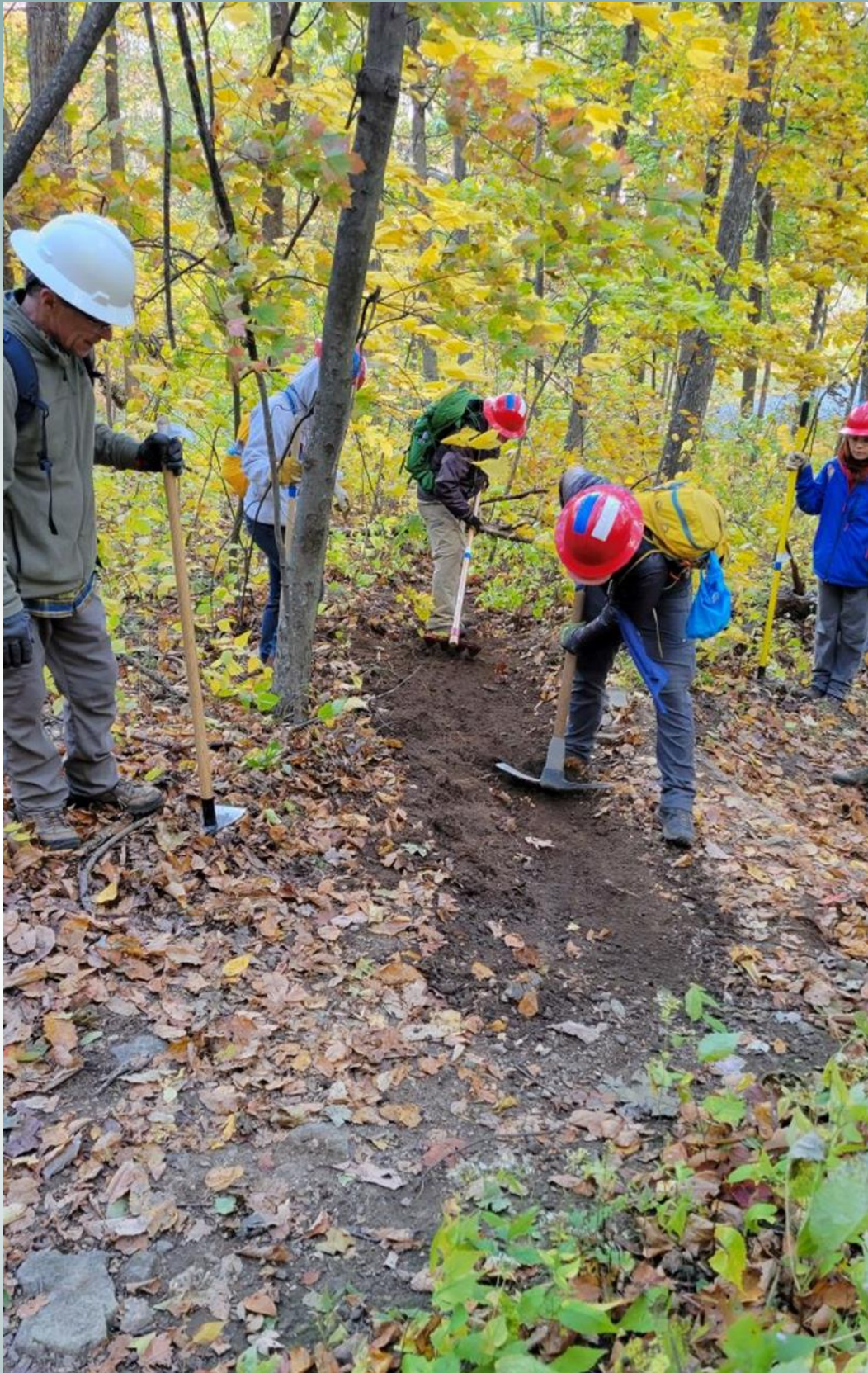
We created a second larger and wider grade dip at a turn in the trail.
