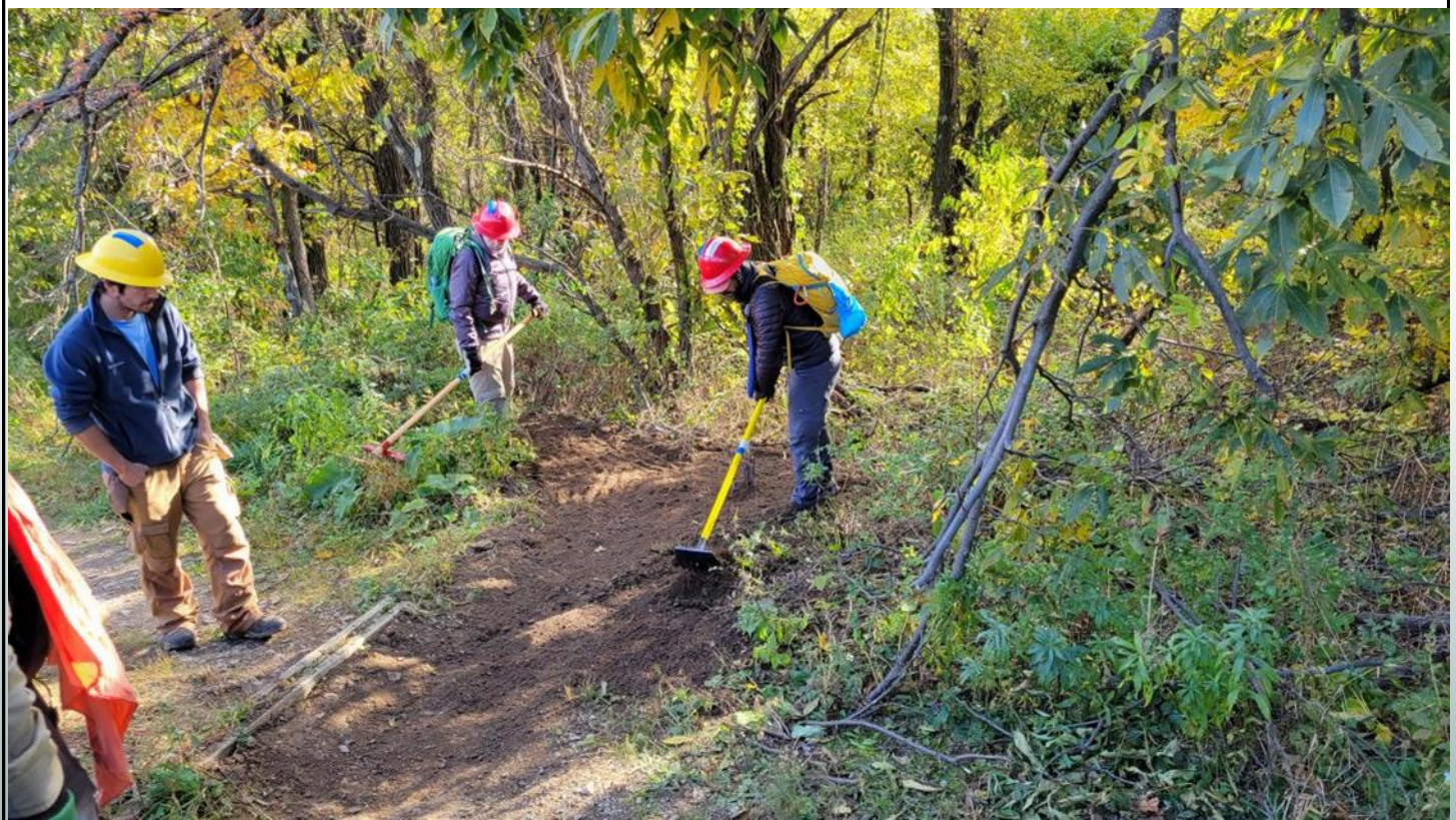
Greg showed us how to create a grade dip or swale. He explained how the running water erodes the trail's tread. The grade dip is easier to install than a water bar and requires less maintenance.
