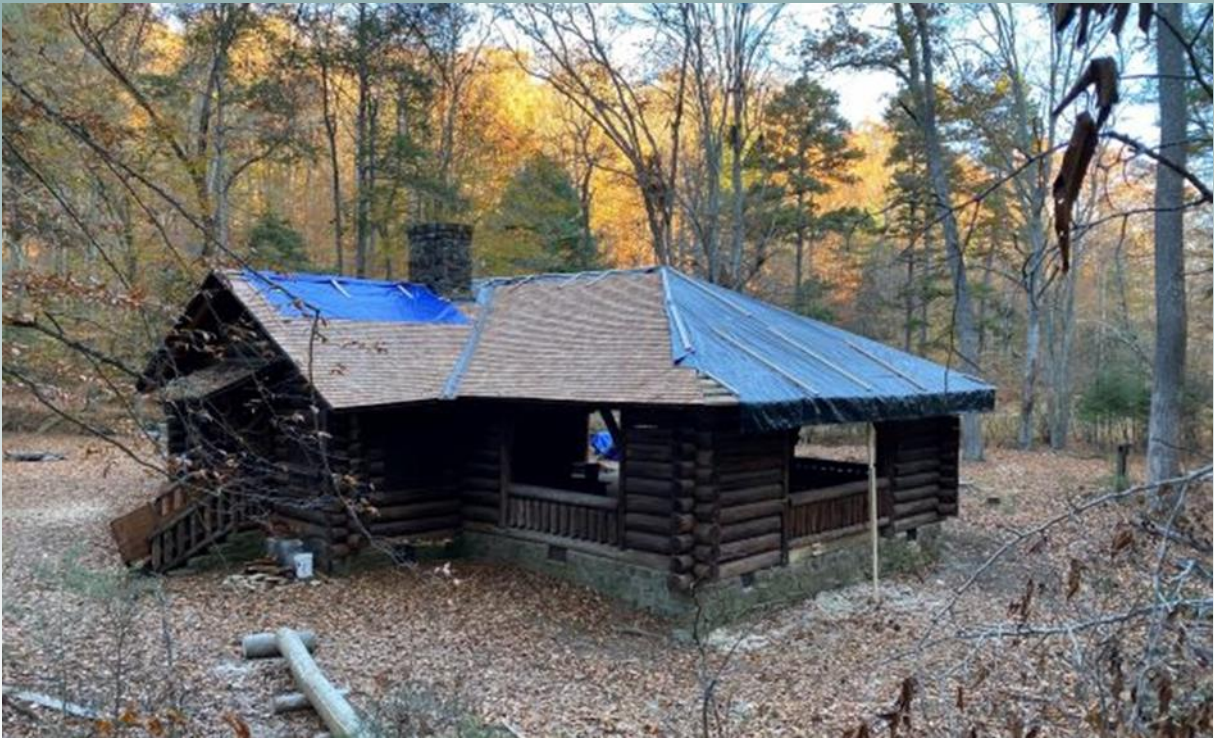
Tarps installed on southwest side.
