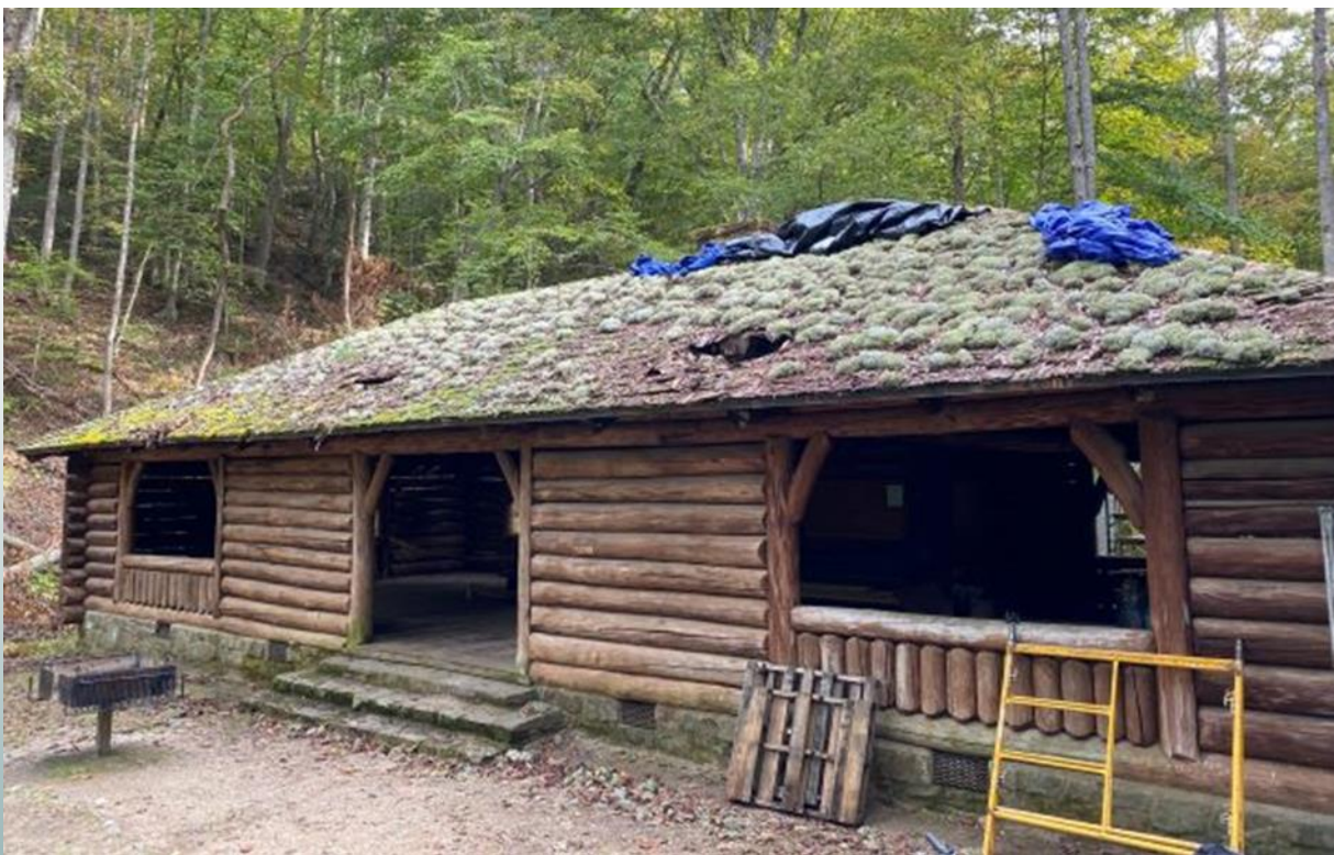
Before starting on the roof repair (early October session).
