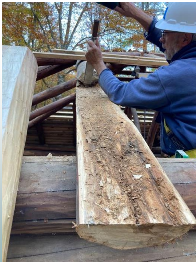
New rafter installation
