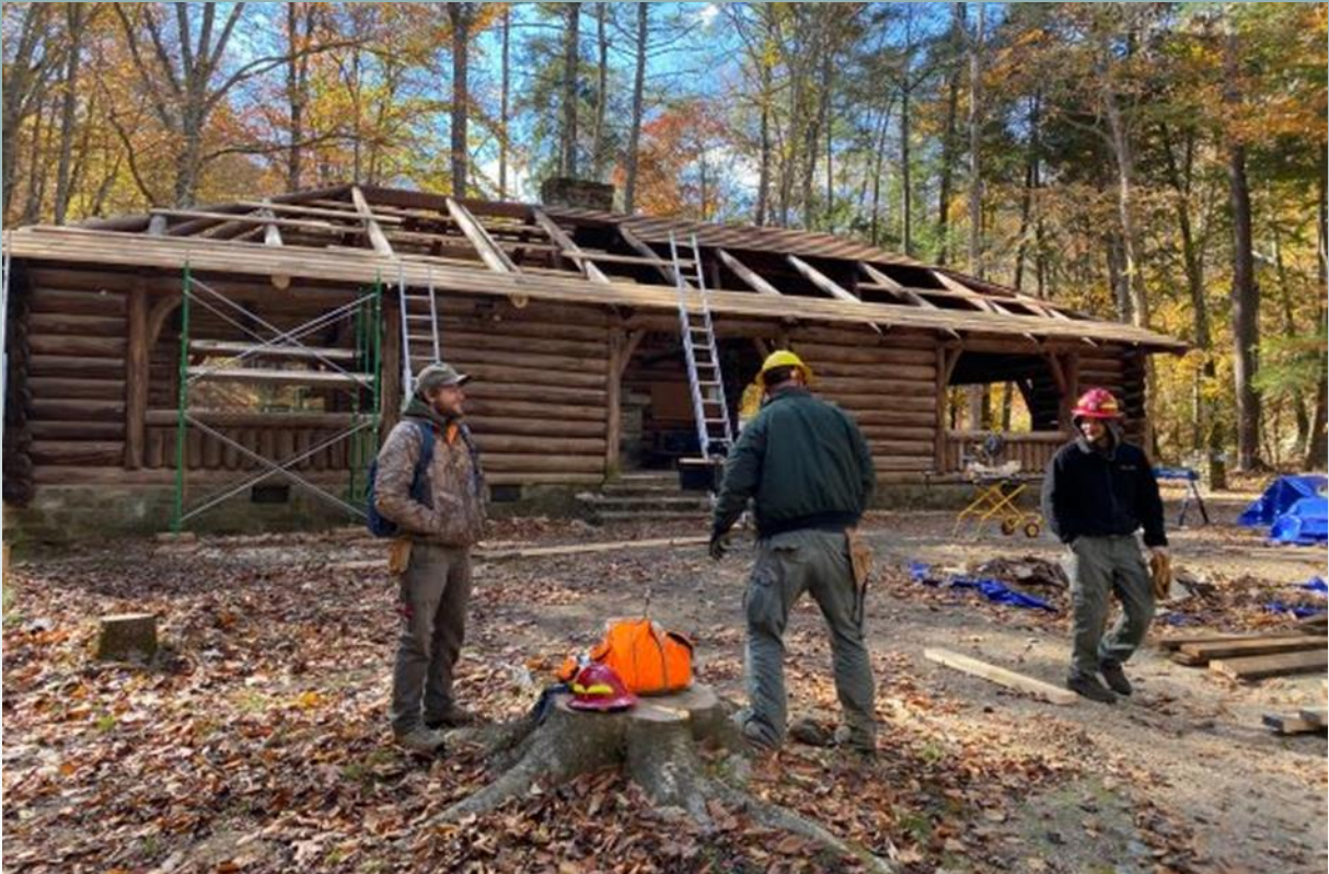
Natural Bridge USFS employees installing new purlins (early November session).
