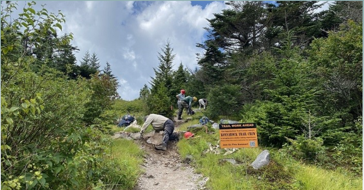
Trail work in progress
