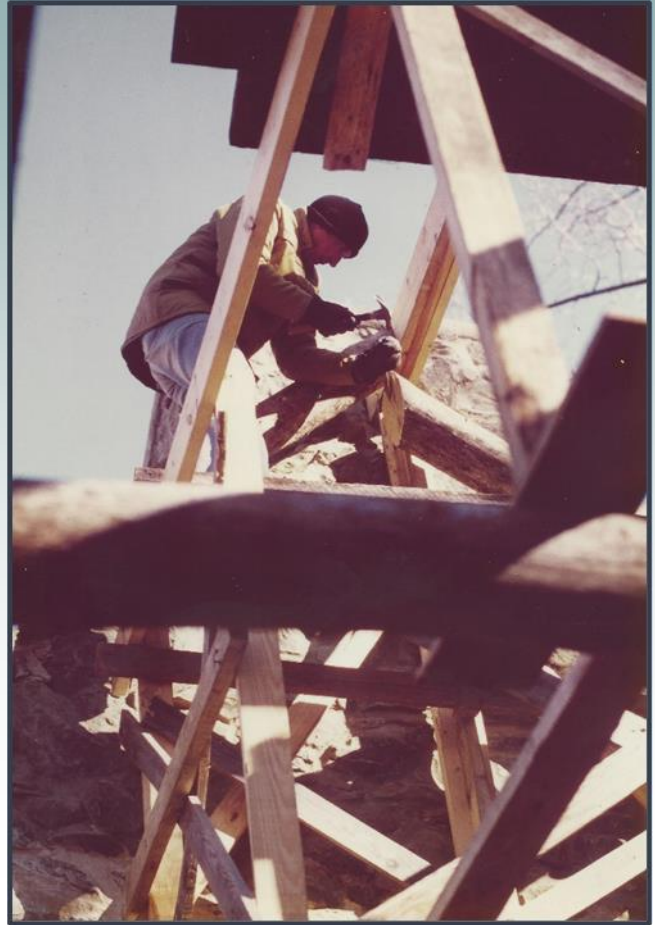
Karl fastening a shutter into place and chiseling the end of the roof rafter
