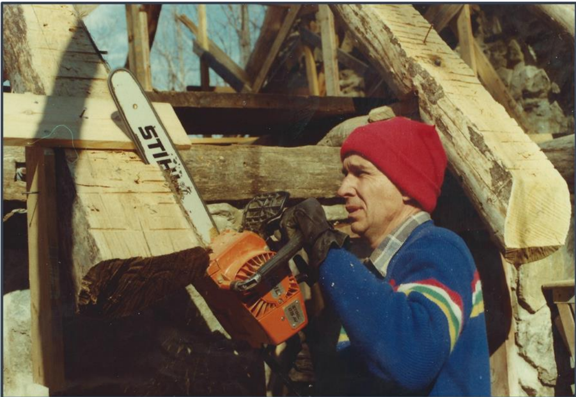
Karl trimming the end of a rafter
