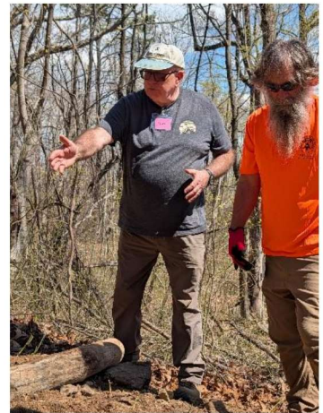
Jim on log waterbar installation
